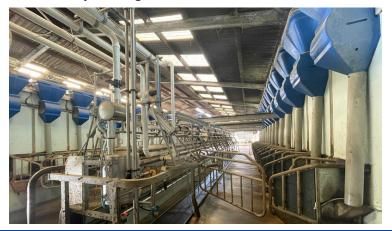
Handling area which comprises of an integral *Dairy Herd Accomodation (Building 2):* with foot trimming crush and race.
